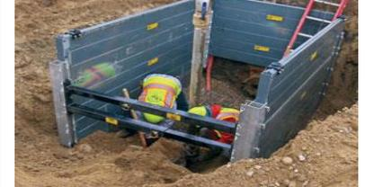
Designing a protective system can be complex because you must consider many factors: soil classification, depth of cut, water content of soil, changes caused by weather or climate, surcharge loads (e.g., spoil, other materials to be used in the trench) and other operations in the vicinity.
