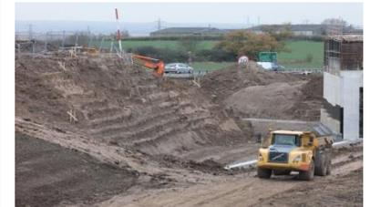
**Sloping** involves cutting back the trench wall at an angle inclined away from the excavation.
