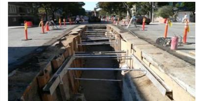
**Shielding** protects workers by using trench boxes or other types of supports to prevent soil cave-ins.
